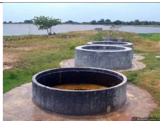
Figure 04: Nelumwewa hot water wells
